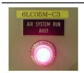
Fig. 4. Equipment Status Lamp
