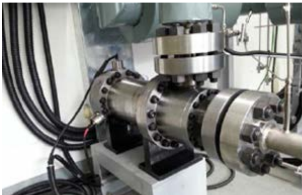
Fig. 2. LP turbine assembly installed in SCIEL [4]
