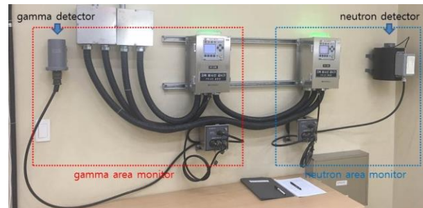
Fig. 1 Gamma area monitor and neutron area monitor installed in the prepare room of radiation controlled area. Basically, the area monitor consists of detector, preamplifier, and rate-meter called the SRM-200.
