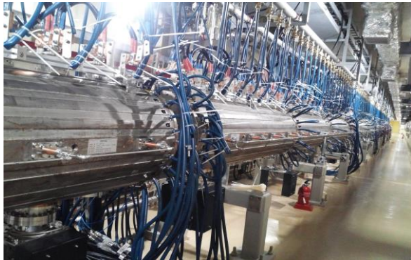
Figure. 1. Accelerator in the tunnel area
