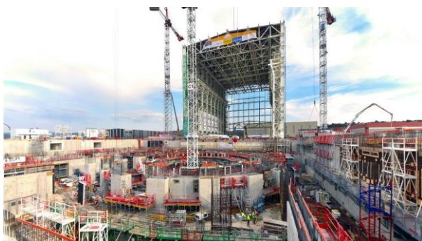
Figure 3 Tokamak complex under construction
