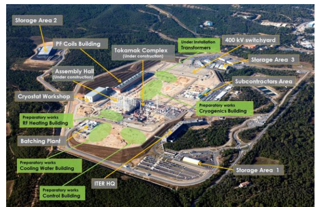
Figure 2 Worksite of ITER construction
