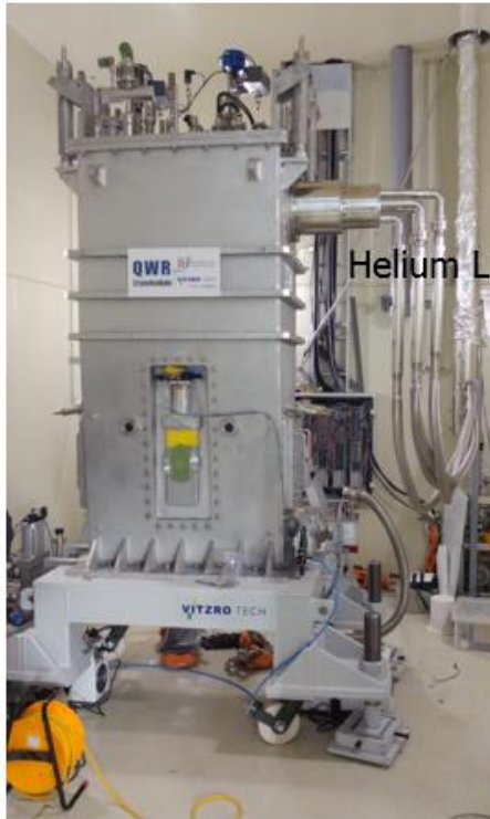
Installed QWR module in Test Bunker
