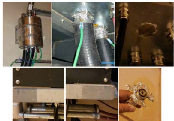
Fig. 3. Reinforcement of ground/cable in the NMS
