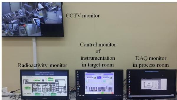
Fig. 3. The installed monitors for the low-flux proton experiments in the control room.
