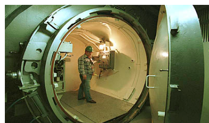
Fig. 3 Airlocks in PHWR
