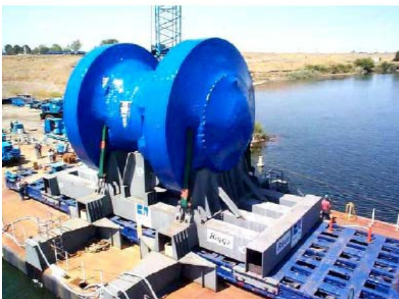
Figure 2. Transportation for reactor vessel of Trojan by Barge
