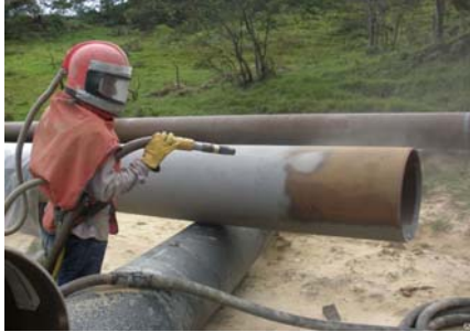
Fig. 3. Abrasive blasting decontamination [3]
