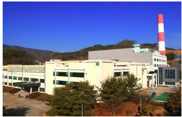
Fig. 1. HANARO after seismic reinforcement
