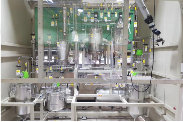
Fig. 3. Full-scale cold mockup of the Mo-99 production system.
