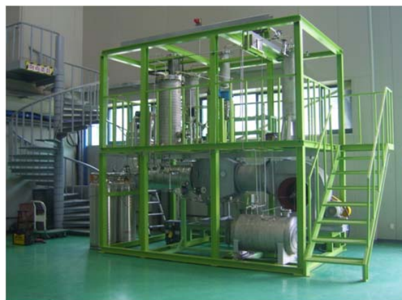
Fig. 2. Photograph of the waste sodium treatment test facility.
