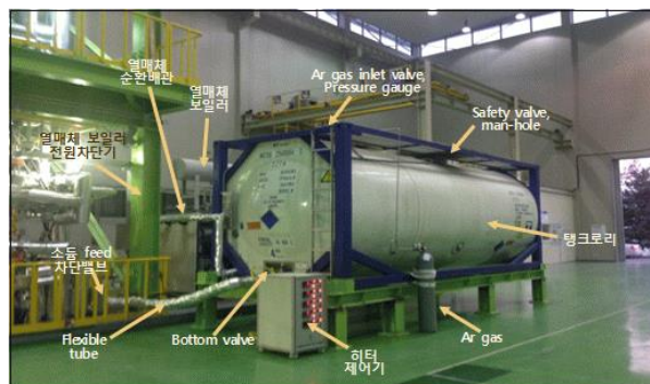
Fig. 3. Example of sodium transfer from ISO tank container to sodium storage tank
