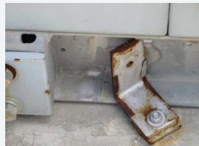
Seismic damage to unanchored cabinets in 2010 Haiti Earthquake
