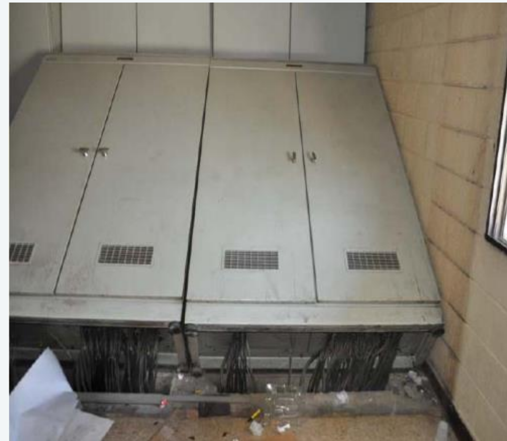
Seismic damage to unanchored cabinets in 2010 Haiti Earthquake
