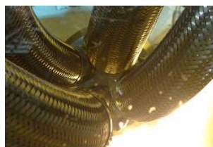
(f) Flexible double pipes
