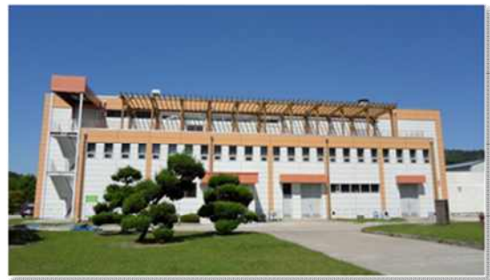
Fig. 2. Front Building View of the PRIDE facility
