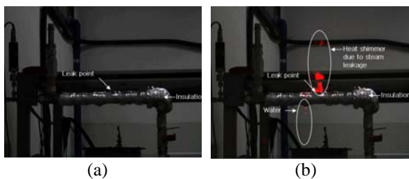
Fig. 3 Experimental result for insulated pipe, (a) Original image, (b) Detected steam by using image signal processing
