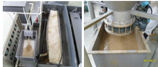
Fig. 5 Soil treatment equipment
