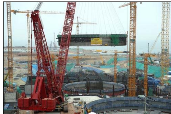
Fig. 11. VHL crane for lifting CLP module in Shin Kori Unit 5 [7].
