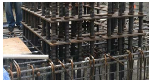
Fig. 8. Template for dowel bar in the basemat [6].
