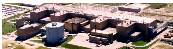
Figure 1 : Industrial low pressure rectangular 'containment' buildings that house 4 reactors in a contiguous volume at the multi unit PHWR station at Bruce. The round building is the vacuum building.
