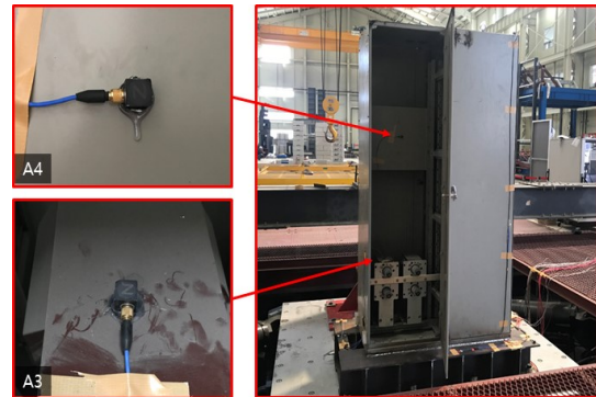
Fig. 3. Location of the Sensor for Acceleration Measurement inside of the Cabinet.
