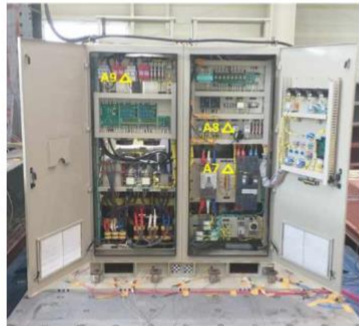
Fig. 3. Implementation of accelerometers (A7, A8, & A9)
