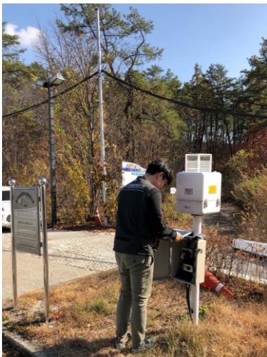
Fig. 5. Control the ERM Cloud Server on Site.
