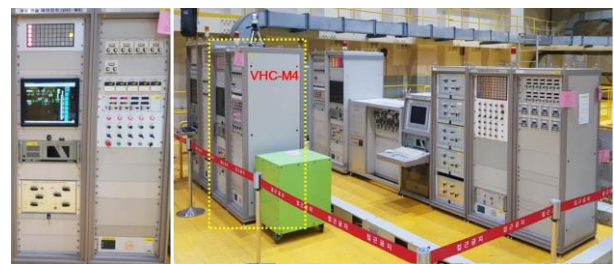
Fig. 6. A new capsule control system (VHC-M4) installed at HANARO for a long-term irradiation
