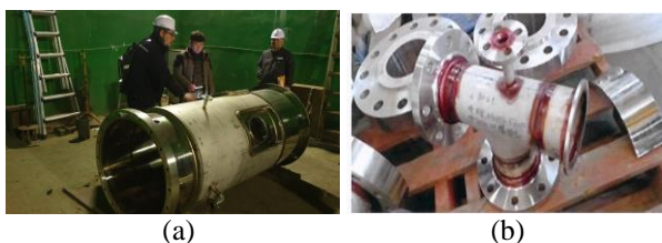
Fig. 4. NDT(Non-destructive testing) ; (a) RT, (b) PT
