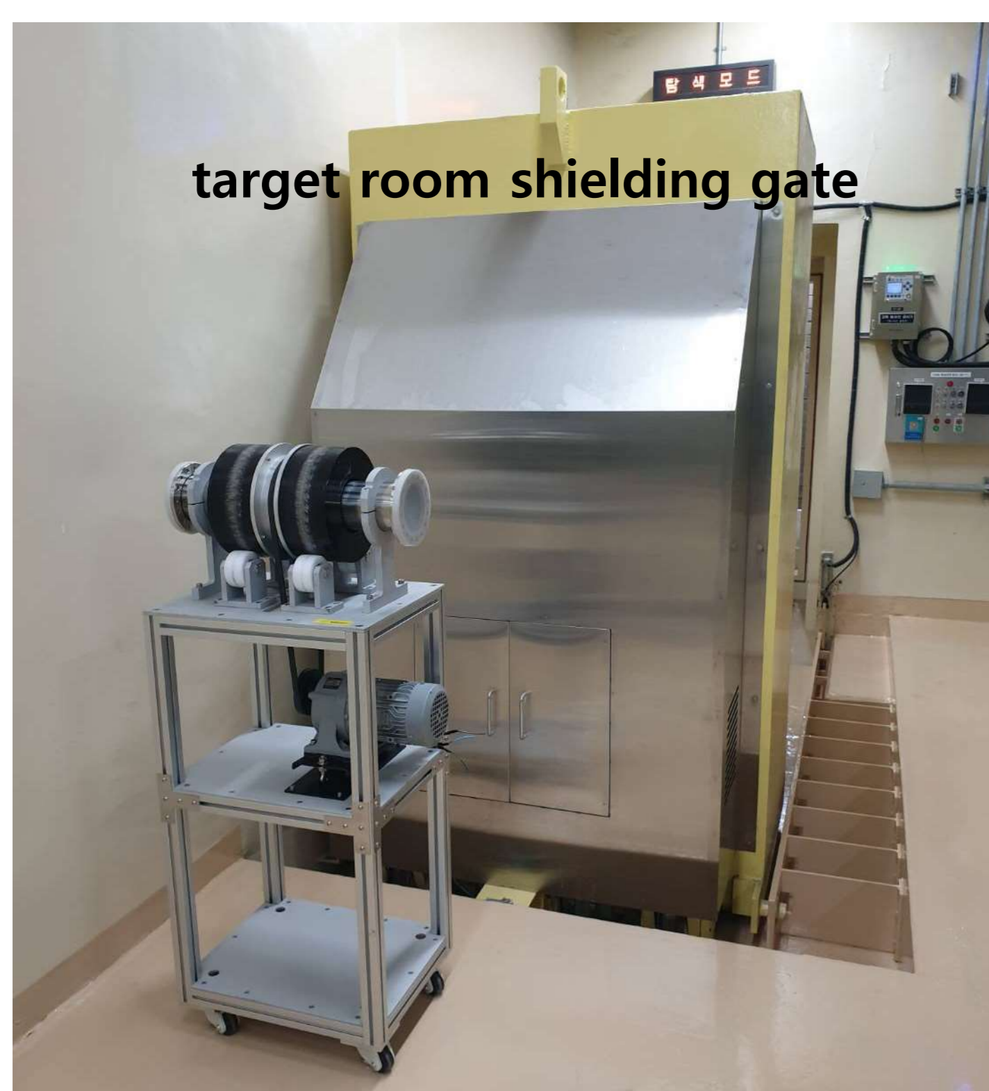
Beam wobbler waiting installation
