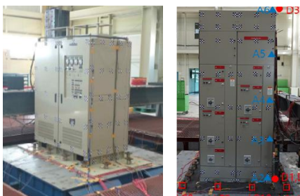
Fig. 1. Test setup of components for shaking table test
