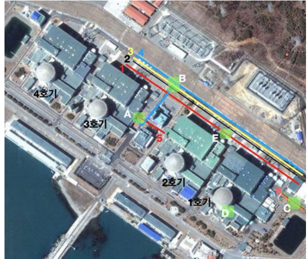
Fig. 4. The buried pipe lines at Wolsong NPP site (by civil investigation team on April 2021 [4]).
