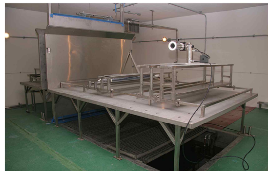
Fig. 1. High-level Gamma-ray irradiation facilities operated by the Advanced Radiation Research Institute of the Korea Atomic Energy Research Institute – 93 sources of cobalt 60 are loaded, with a total radiation dose of 193,611Ci.
