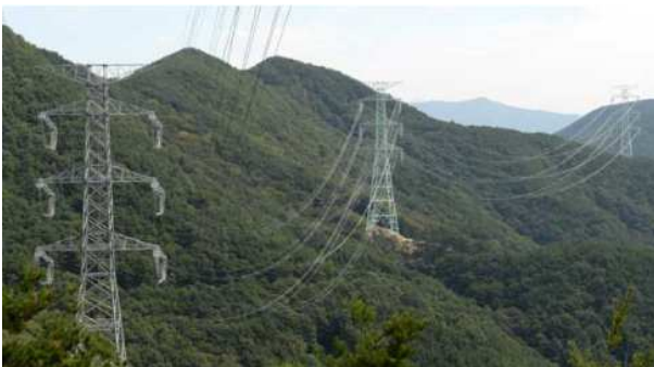
Fig. 1. Towers in mountain slope
