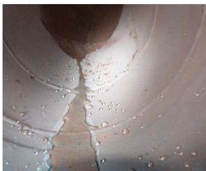
Fig. 3. ODAICON® Application for Layup at Embalse (FW Heater)
