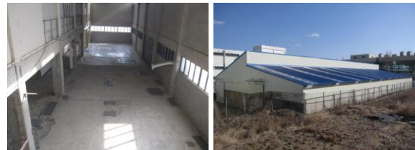
Fig. 2. UCP after decommissioning and remodeled lagoon
