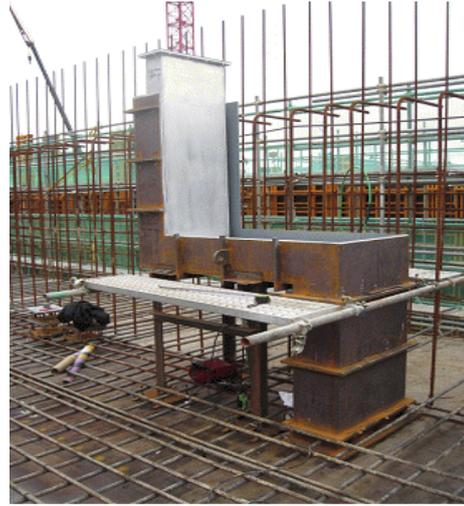
Fig. 6: Installation of waveguide penetration section
