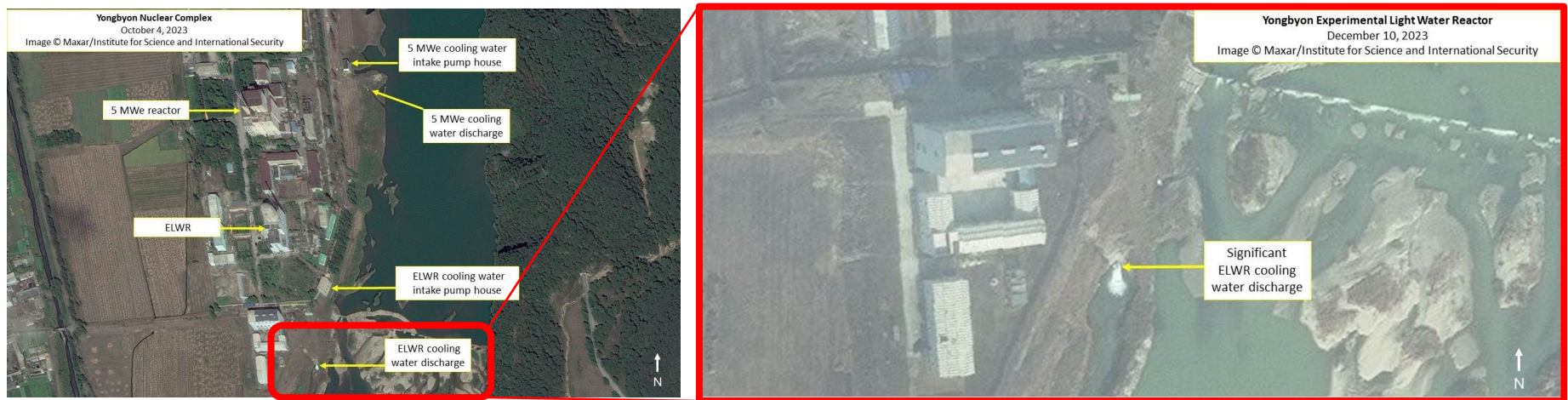
Figure 4. A significant amount of water discharge from the ELWR (Left: October 4, 2023 / Right: December 10, 2023 ) [6]
