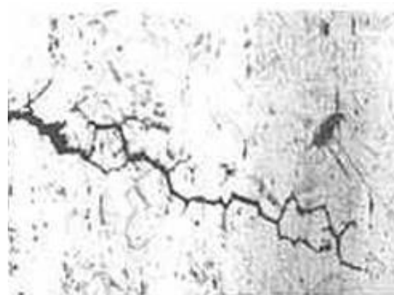
Fig. IASCC crack observed in Baffle bolt [2]
