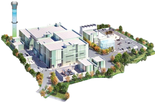
Fig. 1. Plan view of KJRR facility. 154 kV GIS & transformer, electric building, and DG building in north of UB. Cooling tower, demineralized water system, and natural evaporation building in west of RB.
