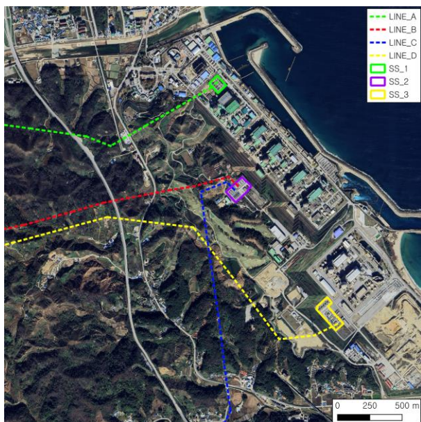
Fig. 2. Offsite power system near the Hanul NPP
