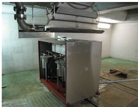
Fig. 2. Reactor for irradiation of transformer oil.
