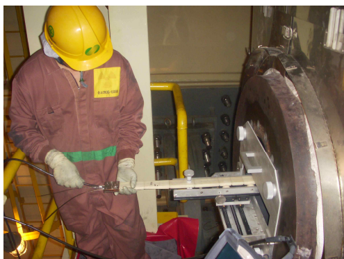
Fig. 4. Operator Inspecting the FDP at Ulchin
