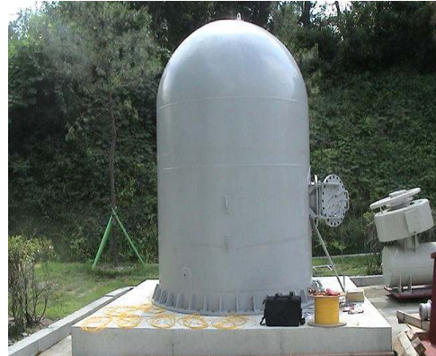
Fig.3. Steel Miniature Containment Structure
