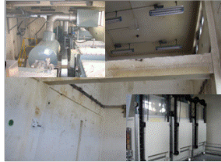
Fig.1. Before and after dismantling of lagoon sludge waste treatment facility
