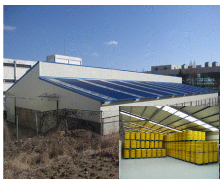
Fig.5. View of lagoon remodeled for use as an interim waste storage facility
