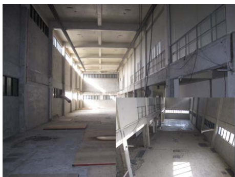
Fig.3. Concrete decontamination of the plant
