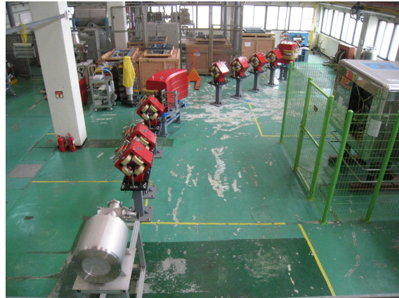
Figure 2: TR104 Beamline for the precedent installation practice at KAERI site
