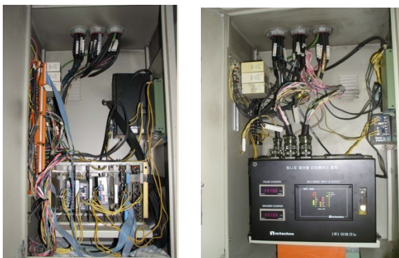
Fig. 5 Before and After the Installation of the Device
