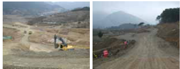
Fig. 6. Photographs of the construction site
