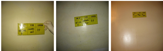
Figure 4. Liner plate, Wall and Floor of Containment Building of Yonggwang Unit 1&2
