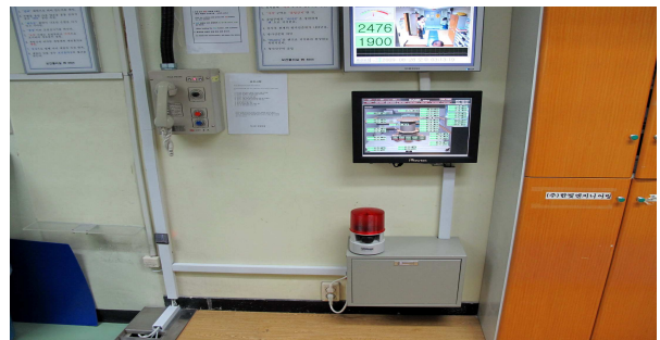
Fig. 6. Installation of voice-flash Alarm and Control PC
