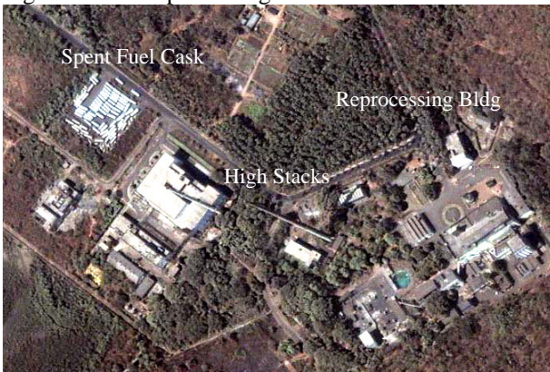
Fig. 2. Indian Reprocessing Plant
